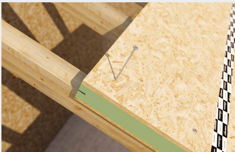
Fastening SIP panels with 8 mm | 0.32 inch diameter TBS screws.
