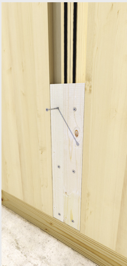
> Fastening CLT walls with 6 mm diameter HBS screws.
