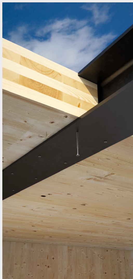
Mixed steel-to-timber structural joint
