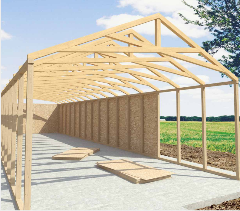
Fastening Wood Trusses outdoors.
