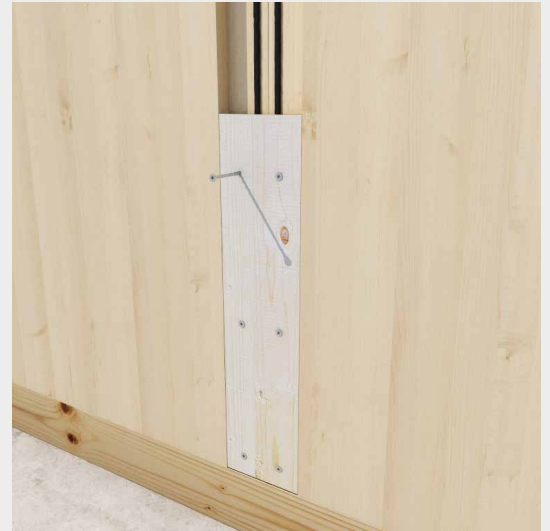
Fastening CLT walls with 6 mm | 0.24 inch diameter HBS screws.
