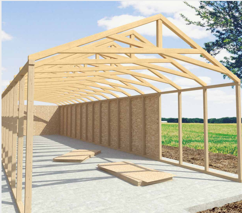
Fastening Wood Trusses outdoors.
