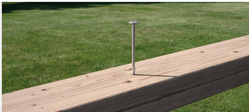
Fastening Wood Trusses outdoors.
