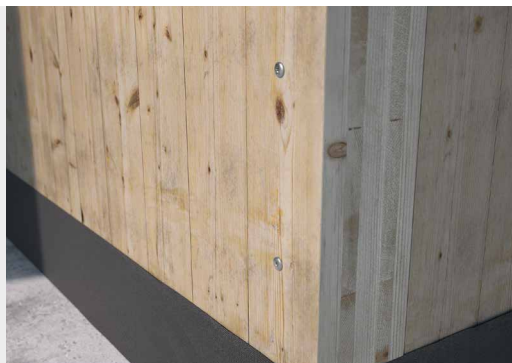
Fastening CLT walls with TBS screws.
