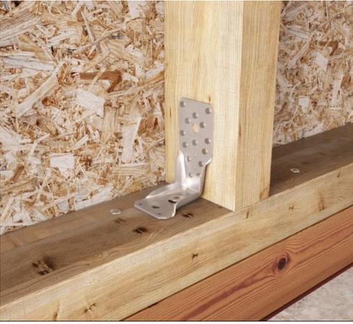
Figure B. 31 Typical installation WKR135
