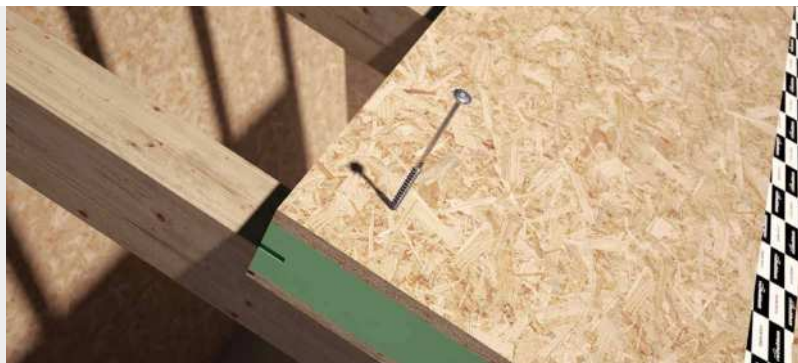
Fastening SIP panels with 0.32 inch (8 mm) diameter TBS screws.
