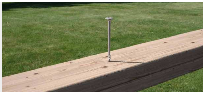
Fastening Wood Trusses outdoors.
