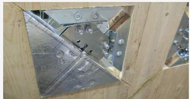
Assembly of the X-SEAL components
