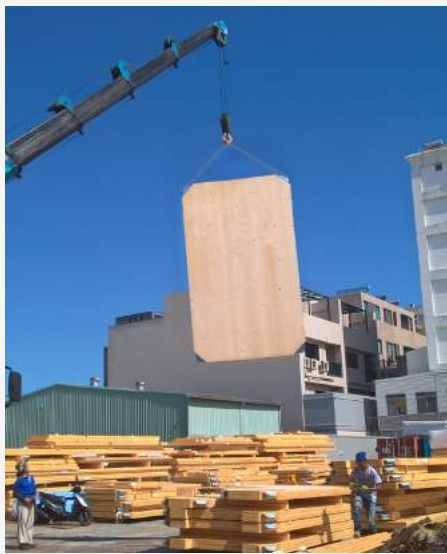
transporting the panels
