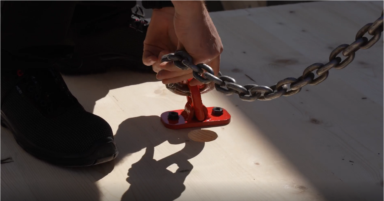
Figure 3. Installing the chain hook on a RAPTOR MINI prior to lifting.
