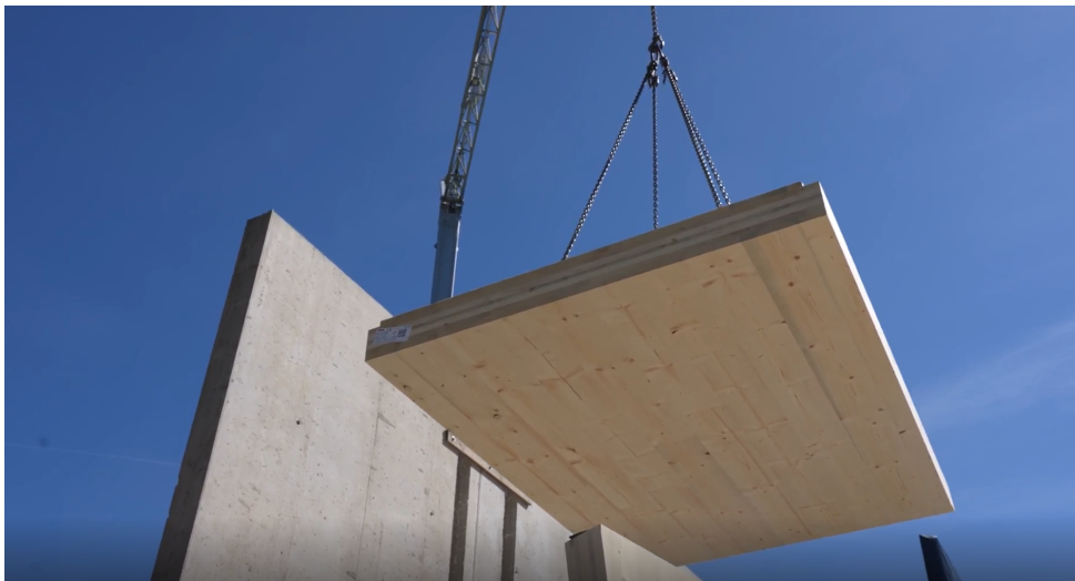
Figure 1. Lifting of a CLT-floor panel on site.
