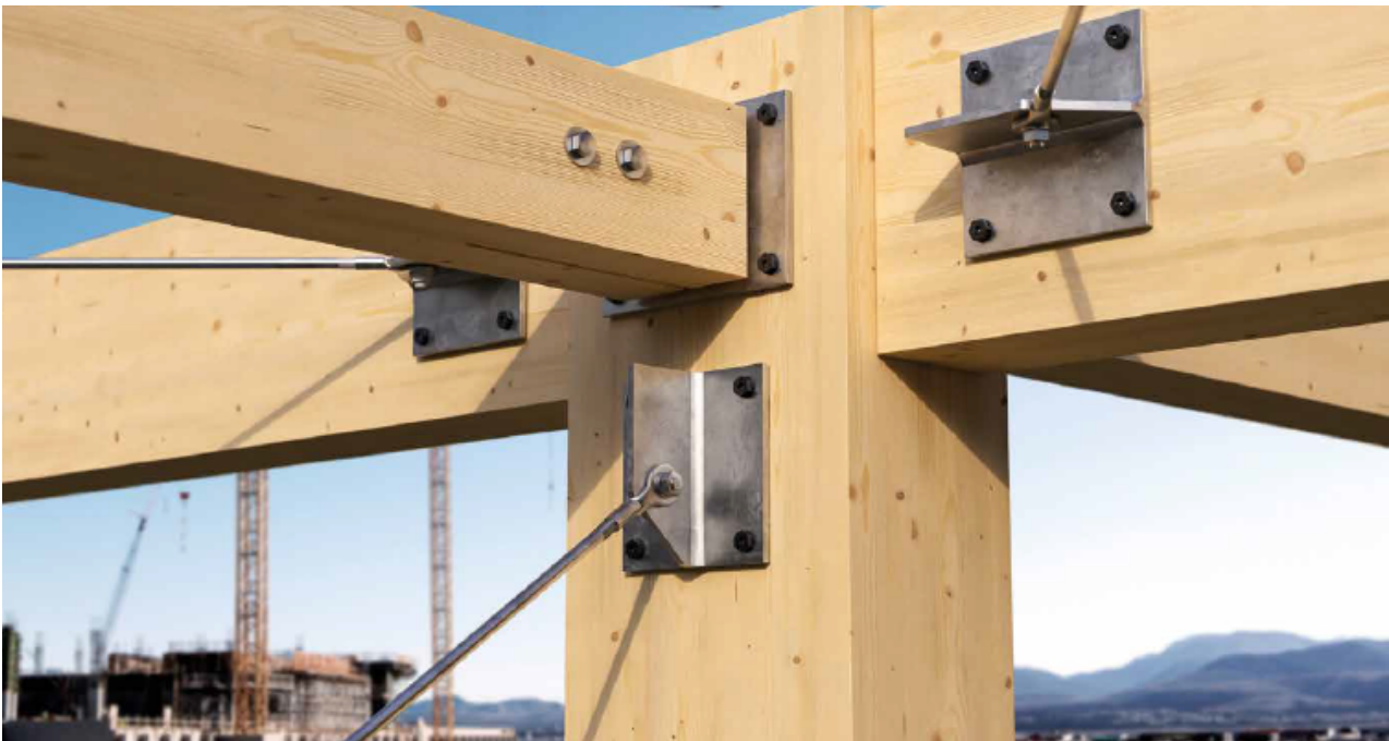
Figure 41. VGS PLATE in a structural application.
