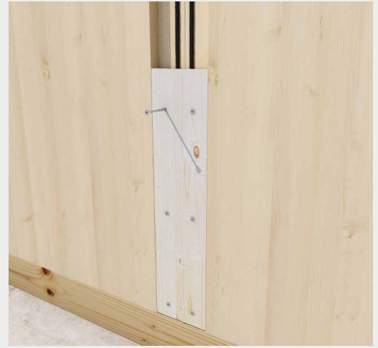
Fastening CLT walls with 6 mm diameter HBS screws.
