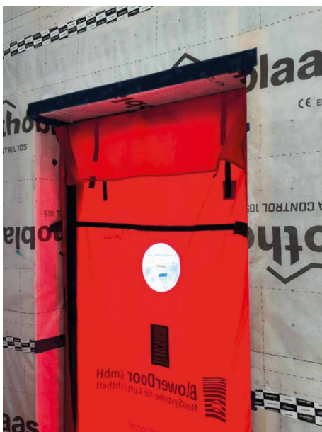
A Blower-Door test carried out at an intermediate stage, are installed before building services and finishes, to verify the continuity of the airtight layer.
