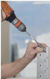
ALUMEGA JVG tightening option 1
