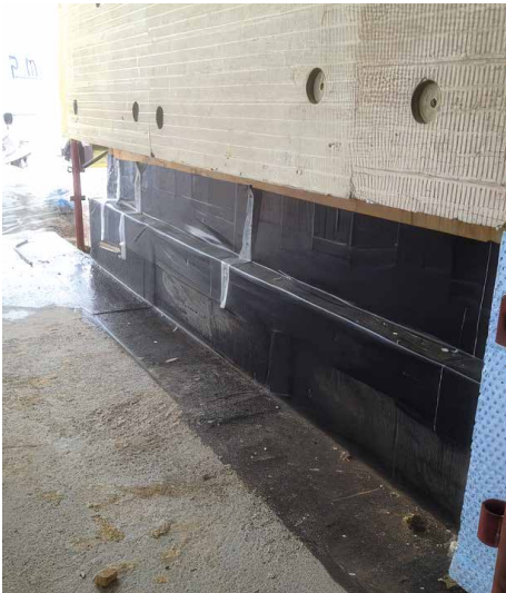
Timber wall raised on a kerb, with moisture-resistant insulation used at the base of the wall.
