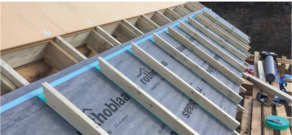
Membrane correctly installed from the bottom up, with layer continuity ensured by tapes and nail sealing.
