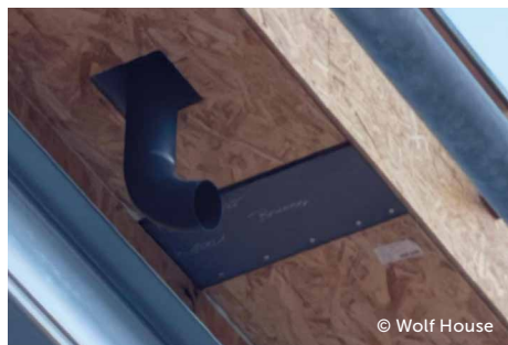
Temporary on-site waterproofing installed correctly.
