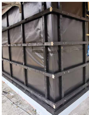
Clean and unobstructed ventilation cavity to promote airflow.
