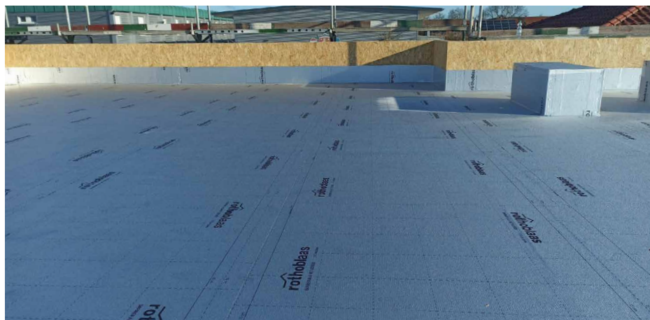
Self-adhesive barrier applied under suitable weather conditions, with continuous installation and correctly executed overlaps.
