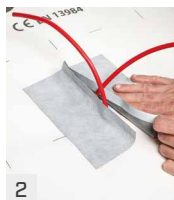
Hot-air sealing.
