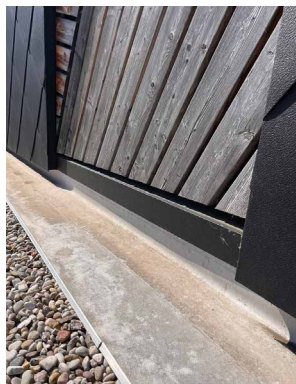
Drainage system at facade breaks/discontinuities.
