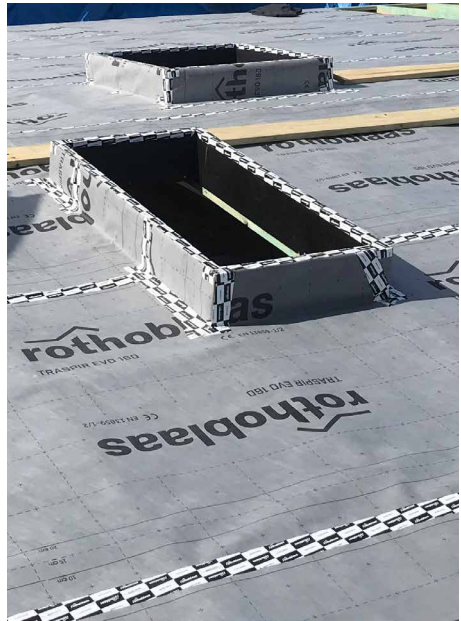
Membrane correctly taped around door and window openings.
