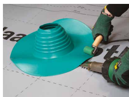
Hot-air sealing.
