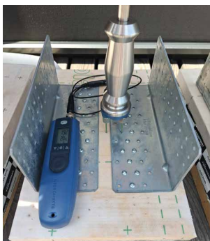
Damage caused by the installation of a plate fastened with screws.
