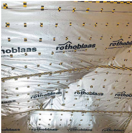
Vapour barrier extensively damaged and repaired only locally, with discontinuous remedial work reducing the effectiveness of the layer.
