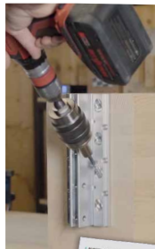
ALUMEGA JVG tightening option 2
