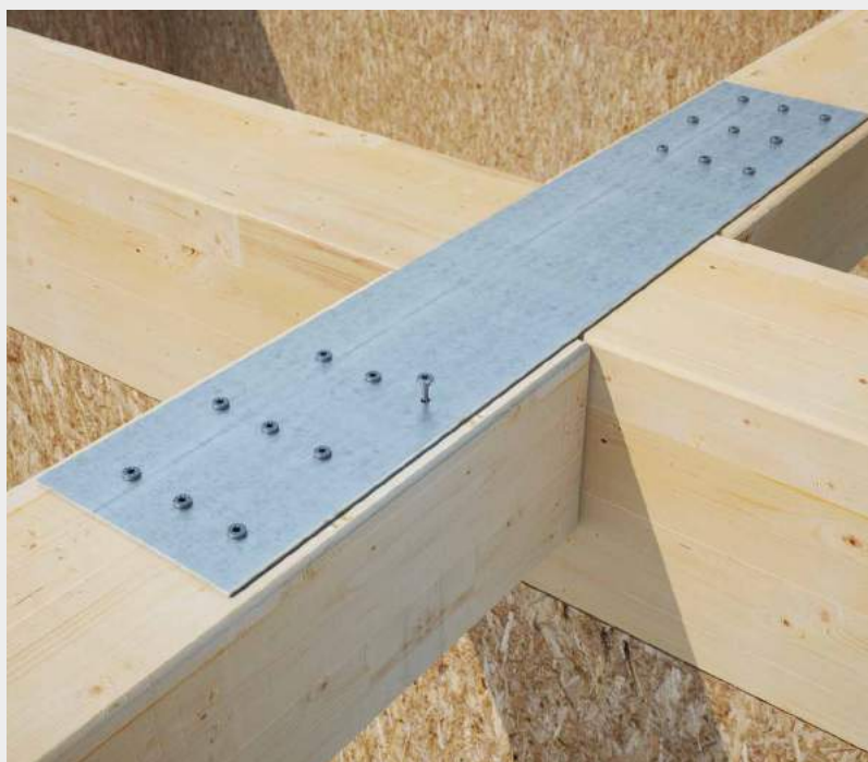
Steel-to-timber shear joint
