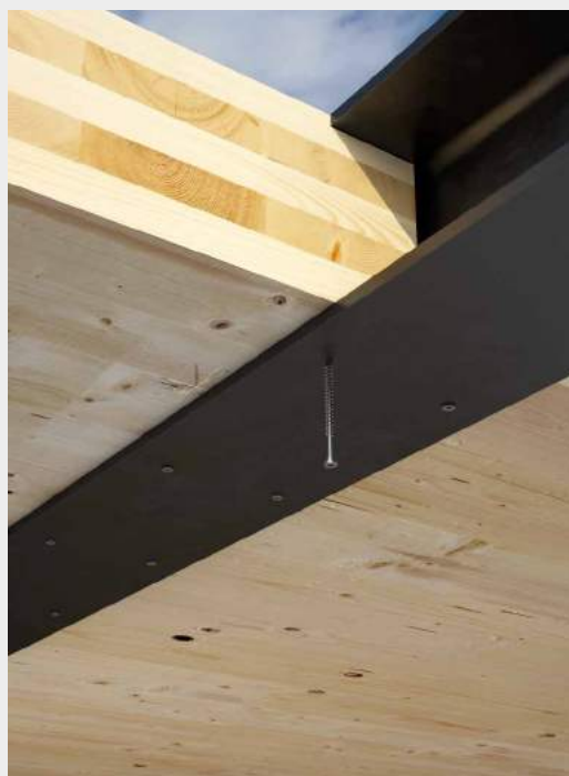
Mixed steel-to-timber structural joint
