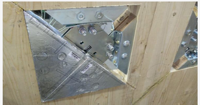
Assembly of the X-SEAL components
