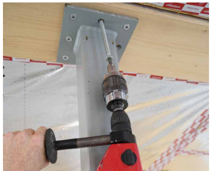
During tightening, the TORQUE LIMITER disengages at the set torque value.
